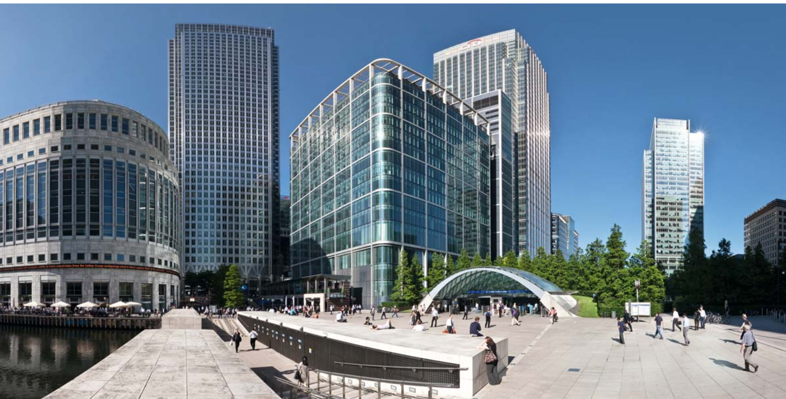
Canary Wharf, London, UK: JORDAHL supplied JTA anchor channels for the façade connection – Photo by David Iliff
