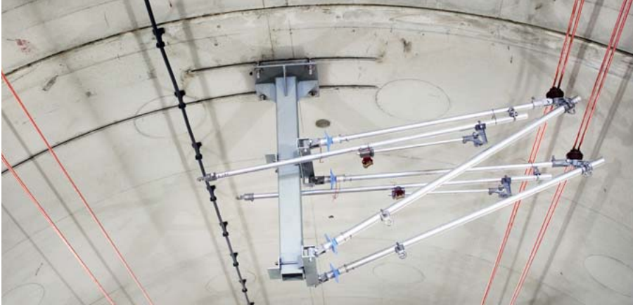
Curved anchor channel pair for safe fastening of catenaries in railway tunnels
