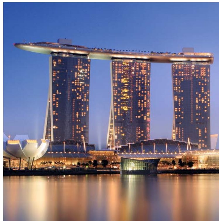
Marina Bay Sands Resort & Casino, Singapore: JORDAHL® anchor channels for fastening the glass façade elements – Photo by Stefano
